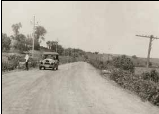
Dirt Lincoln Highway route four miles south of Logan
