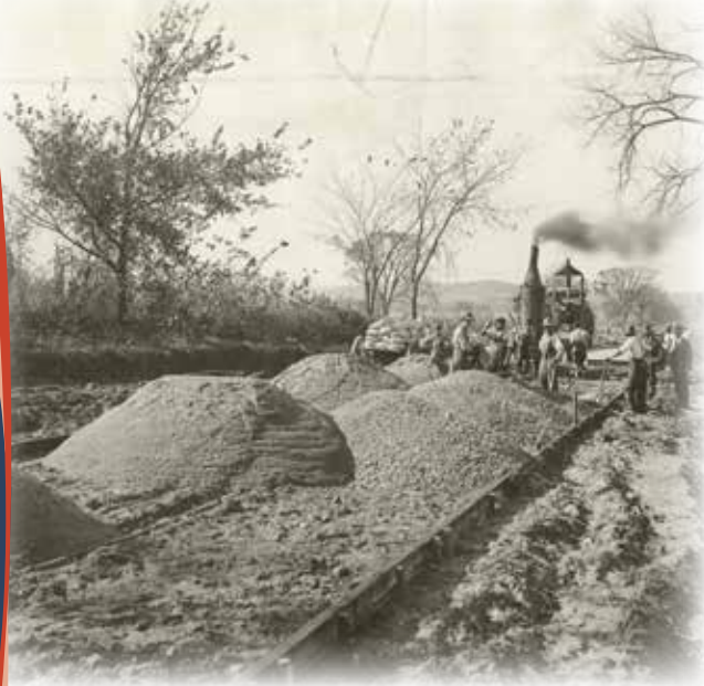
Concrete construction underway in central Iowa, 1915
