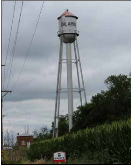
Calamus water tower
