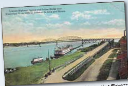
This circa 1915 postcard shows how the truss bridge made a 90-degree turn as it approached Lyons, where you're standing. Lyons became part of Clinton in 1897.
