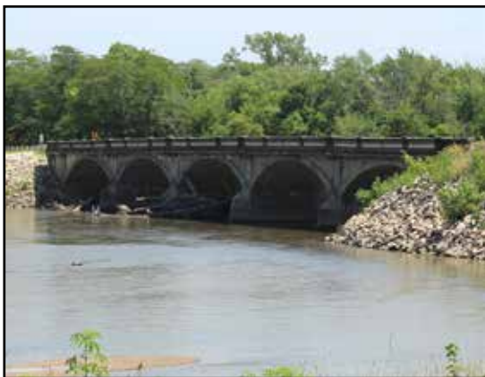
1913 Eureka Arch Bridge over the Raccoon River
