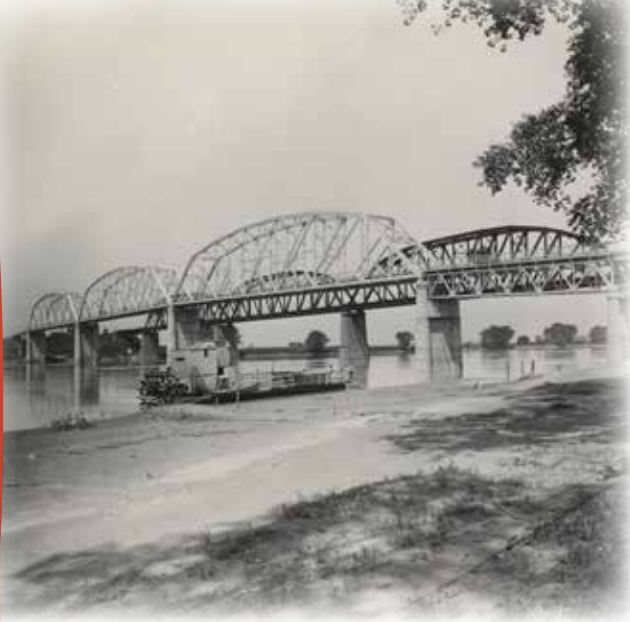
1929 Abraham Lincoln Memorial Bridge that once crossed the Missouri River from Iowa to Blair, Nebraska
