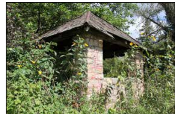
Meskwaki Stone Well House
