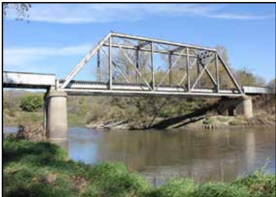
Railroad bridge over the Boyer River near Denison
