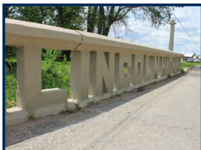
Tama's E. 5th St. Bridge
