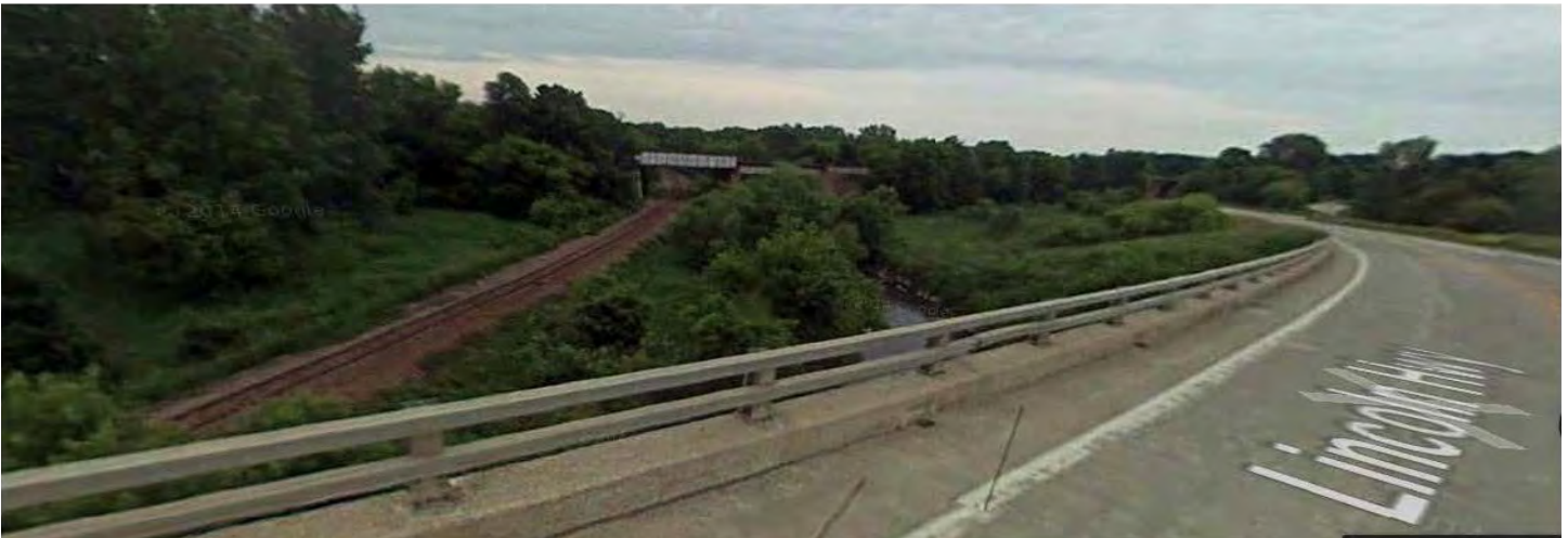
Overpass, looking east
