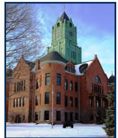
Clinton County Courthouse
