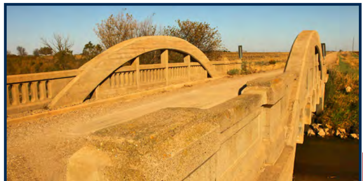
Original Lincoln Highway bridge outside of Beaver in Greene County
