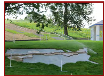
Photo from construction of the Harrison County Welcome Center
