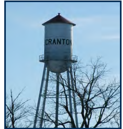
Scranton Water Tower
