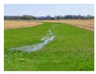
Grassed waterways are constructed graded channels that are seeded to grass or other suitable vegetation. The vegetation slows the water and the grassed waterway
