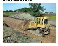
Denitrifying bioreactors move water through a woodchip-filled trench. Bacteria that live in the woodchips convert nitrate runoff into nitrogen gas. Bioreactors
