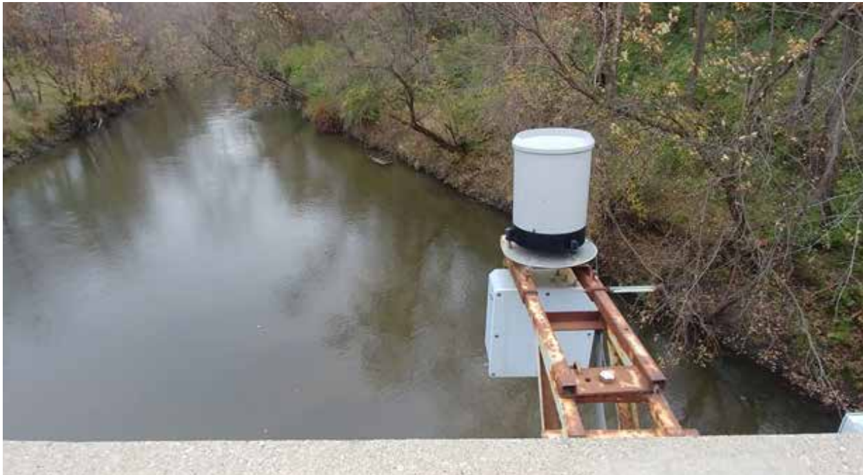
Figure 14: Bridge-mounted stage sensor (City of Ames) on Ioway Creek
